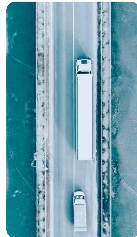
New environmental services are in place
